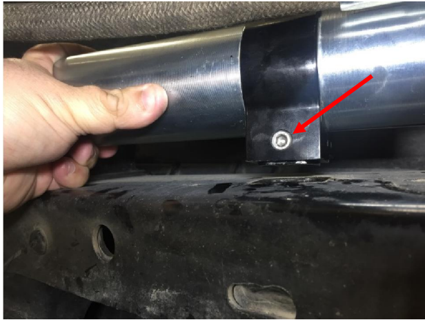
Looking from underside of the frame rail
